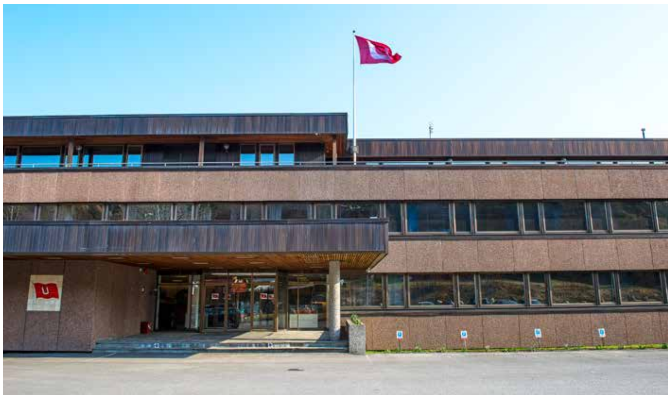
Ugland office building in Vikkilen, Grimstad
